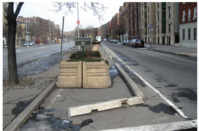
In 2011, prior to Capital project, medians on Grand Concourse were in disrepair: Bronx
