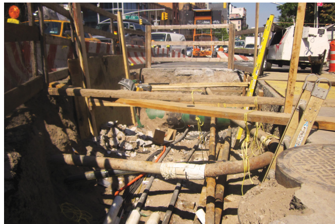
Pipe installation as part of street reconstruction. Capital projects can impact sub-surface conditions and are more comprehensive. They are managed by DDC: Second Avenue and E Houston Street, Manhattan
