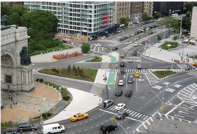
Operational projects usually do not involve sub-surface utility work, drainage, or roadway grading, and they are designed by DOT staff and built either by agency personnel or by a DOT contractor: Grand Army Plaza, Brooklyn
