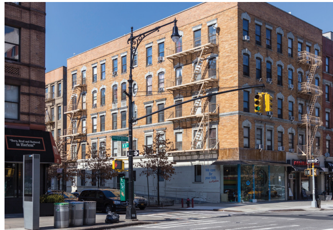
Type M-2A signal pole with Type M pole and Teardrop luminaire (Historic): 114th Street, Manhattan
