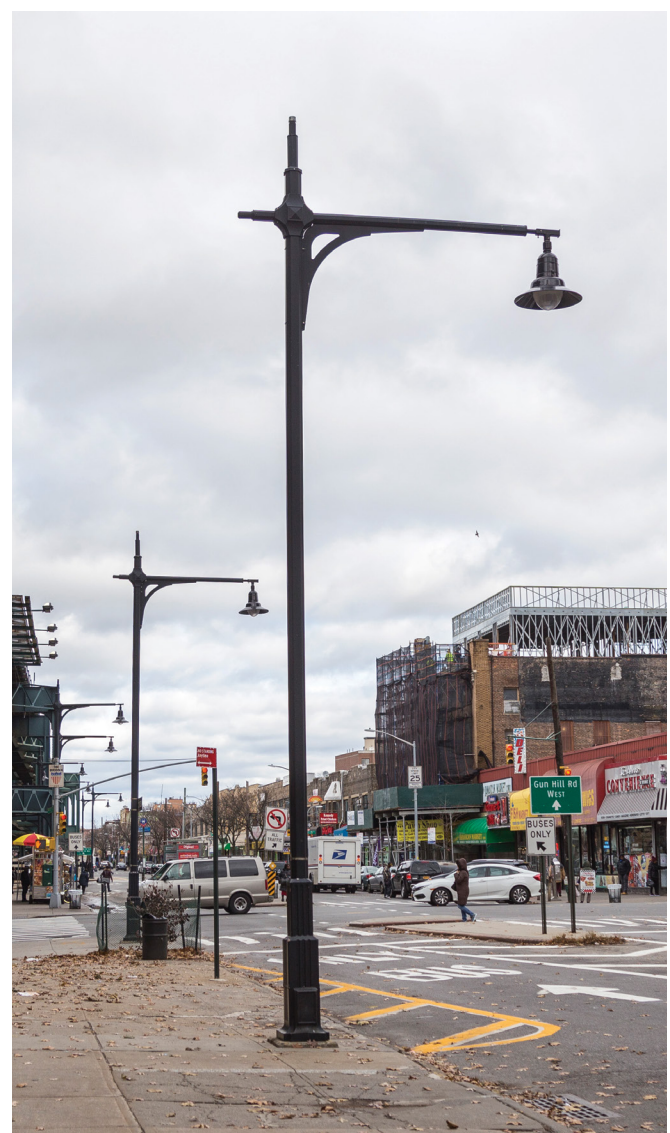
Pole with Shielded Teardrop luminaire: White Plains Road, Bronx
