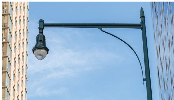
Pole with Teardrop luminaire: Flatbush Avenue, Brooklyn
