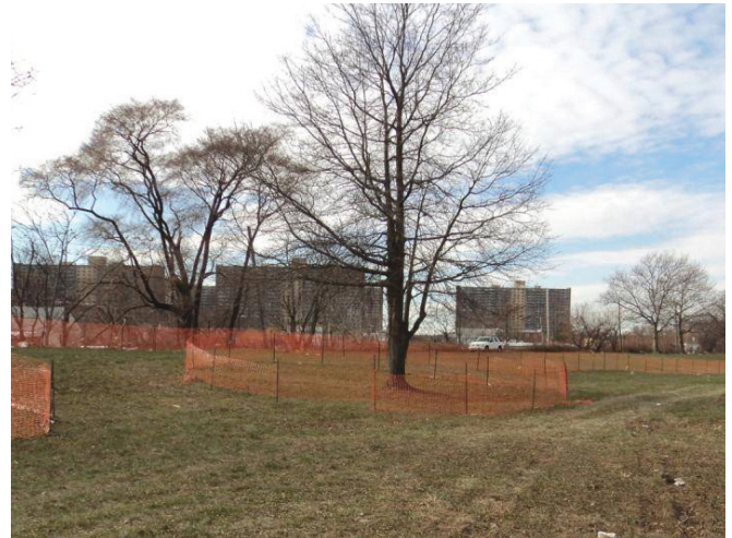
Typical tree protection area (TPA) in a landscape setting; specialized treatments should be used in urban settings: Conduit Avenue, Queens
