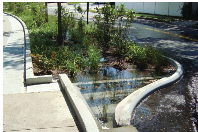
Water can be collected in a forebay, such as the triangular area shown above. This allows sediment and debris to settle before the water continues to the planting area: Westbourne Avenue and Bay 25th Street, Queens (Credit: Parks)
