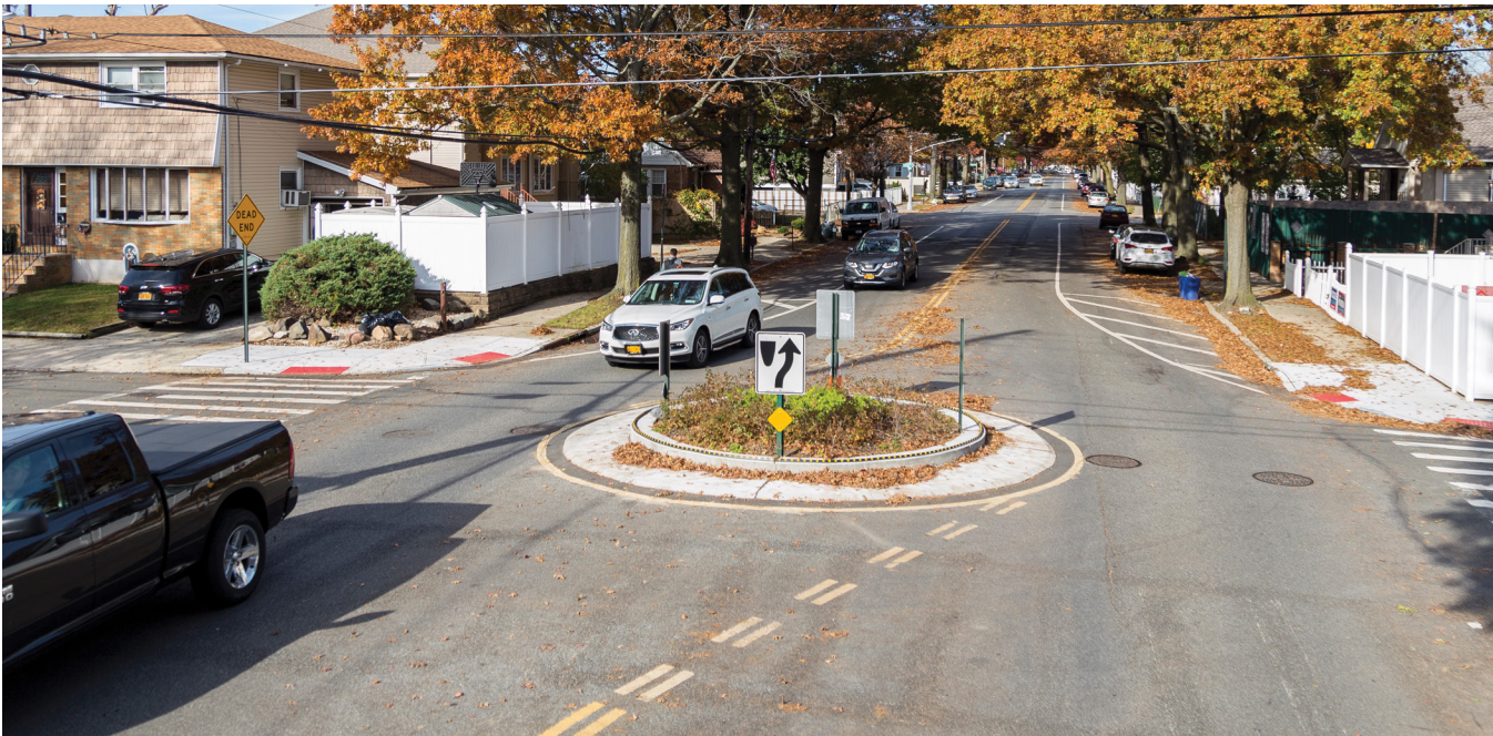
Greeley Avenue and Freeborn Street, Staten Island
