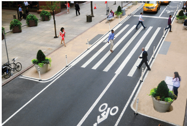
Interim mid-block narrowing at Midtown Arcades: W 51st Street, Manhattan
