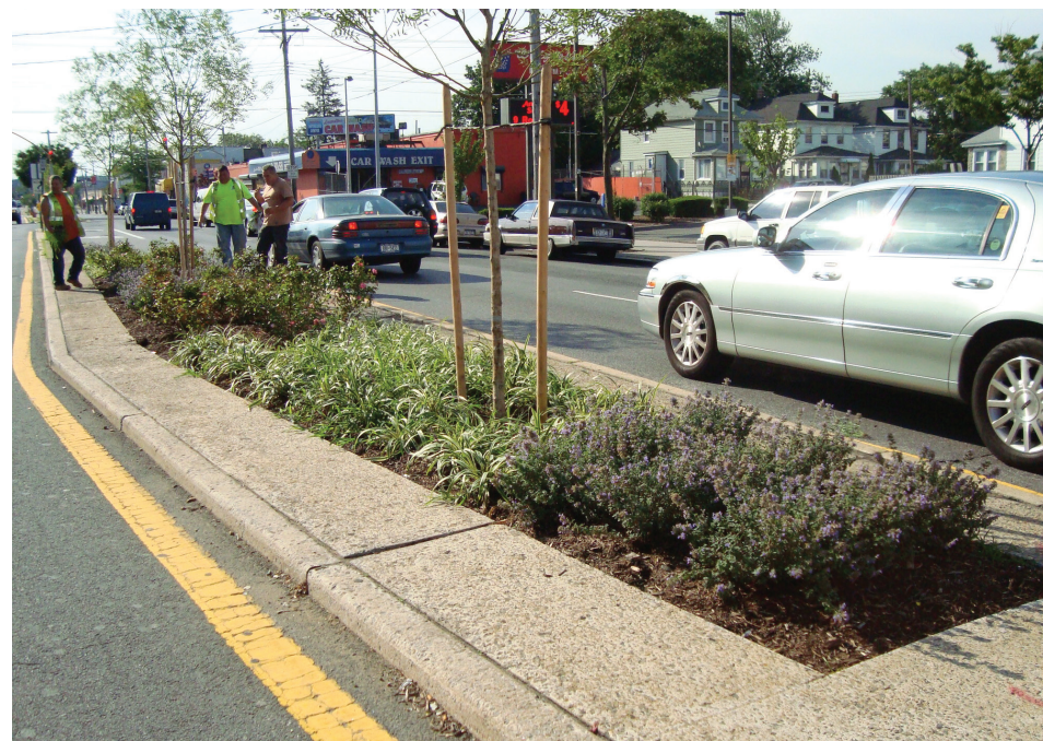
Curb-height median with plantings set back from the curb to allow for easier maintenance: Merrick Boulevard, Queens (Credit: DPR)
