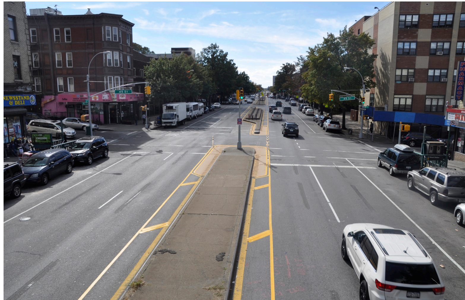
Existing Condition, 4th Avenue
