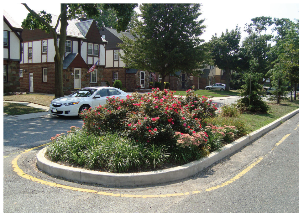
Planted curb-height median: 253rd Street and 86th Avenue, Queens (Credit: DPR)
