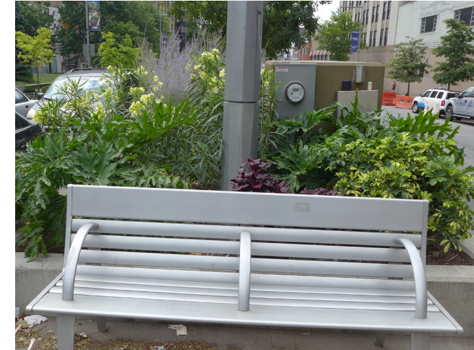
Bench, light pole and RPZ equipment at an intersection along Flatbush Avenue
