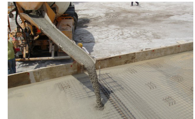
Self-consolidating concrete (Source: Nicolia ready-Mix)
