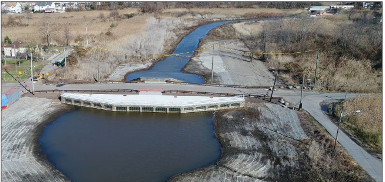
Figure 6 - A DEP bluebelt under construction in Staten Island designed to alleviate chronic flooding. Photo courtesy of JR CRUZ Corp.
